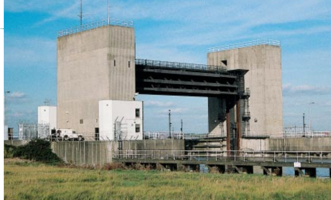
Dartford Barrier from upstream
